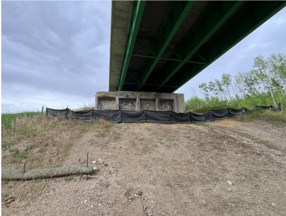
Photo 5 - Looking west at headslope below Abutment 1. Erosion control measures installed in 2023.
