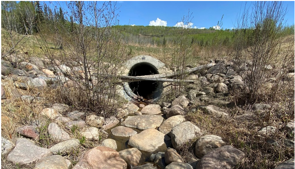
Photo 4 – Looking southeast at culvert inlet.
