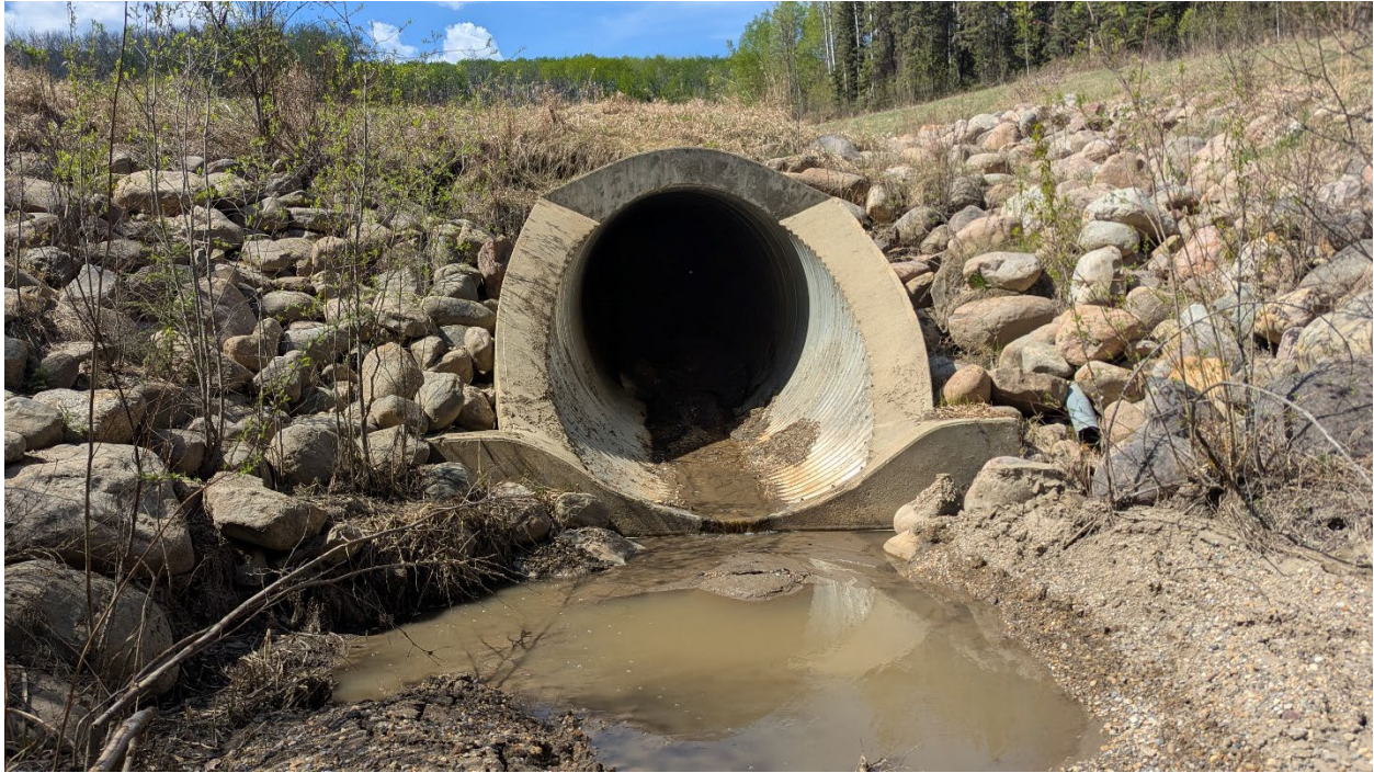
Photo 3 – Looking northwest at culvert outlet.
