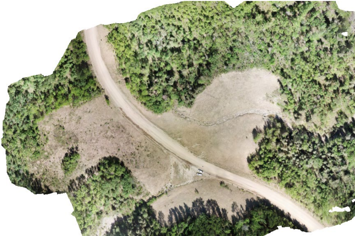
UAV 2023 Orthomosaic: Seepage can be seen along the left side of the highway; the eroding and slumping channel is to the right of the highway.
