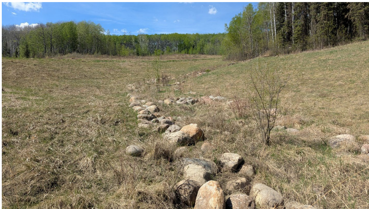
Photo 5 – Looking north at swale near the culvert outlet.
