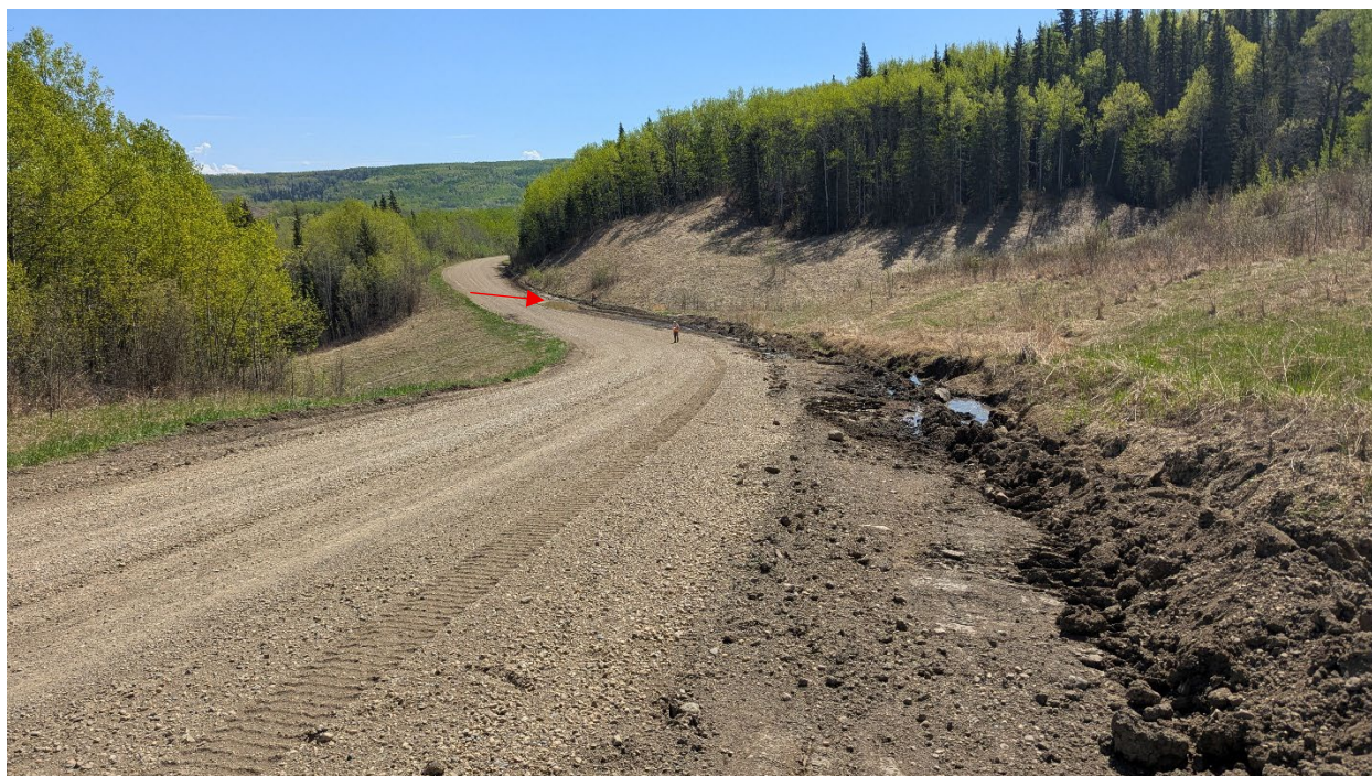
Photo 6 – Looking southwest at road and seepage along west ditch. Note exposed subgrade at edge of roadway and ponded water in the distance (red arrow).
