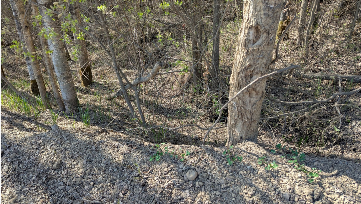
Site 2, Photo 3 – Looking south where scarp continues on the west side of the highway.
