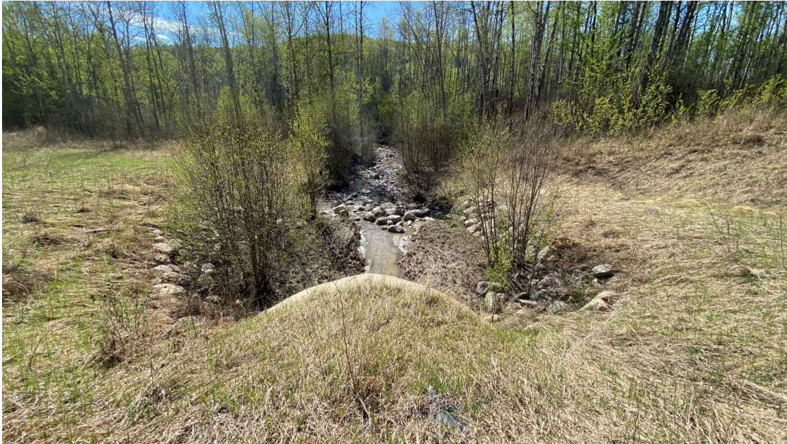
Site 1, Photo 5 – Looking south at culvert outlet. Much of the riprap has been displaced downstream and the accumulated sediment noted in 2023 at the outlet of the culvert has been washed away.
