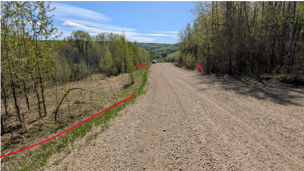
Site 2, Photo 4 – Looking southeast from north end of the site at the sag in the highway where it crosses the slide mass. The visible scarps are shown with red lines.
