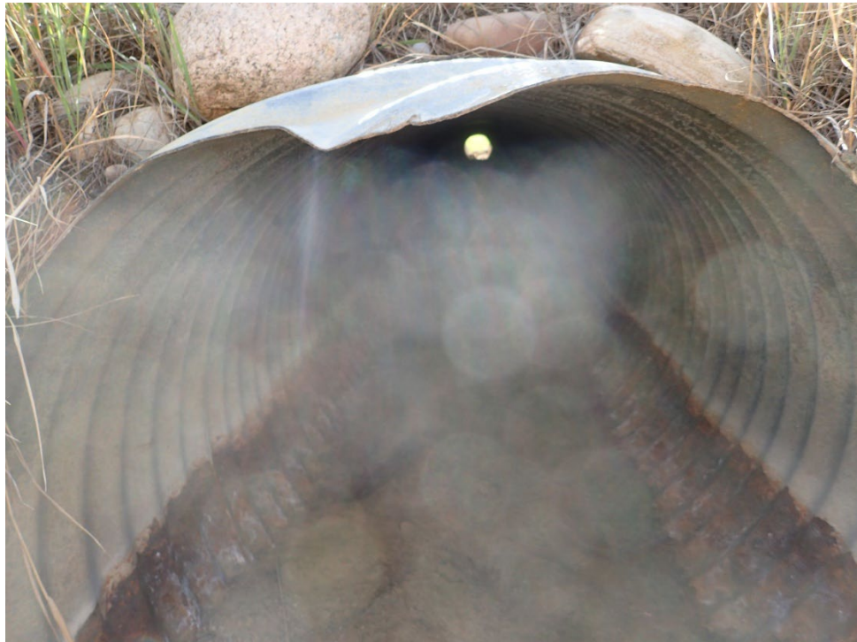
Photo 18 – Looking east at culvert outlet.
