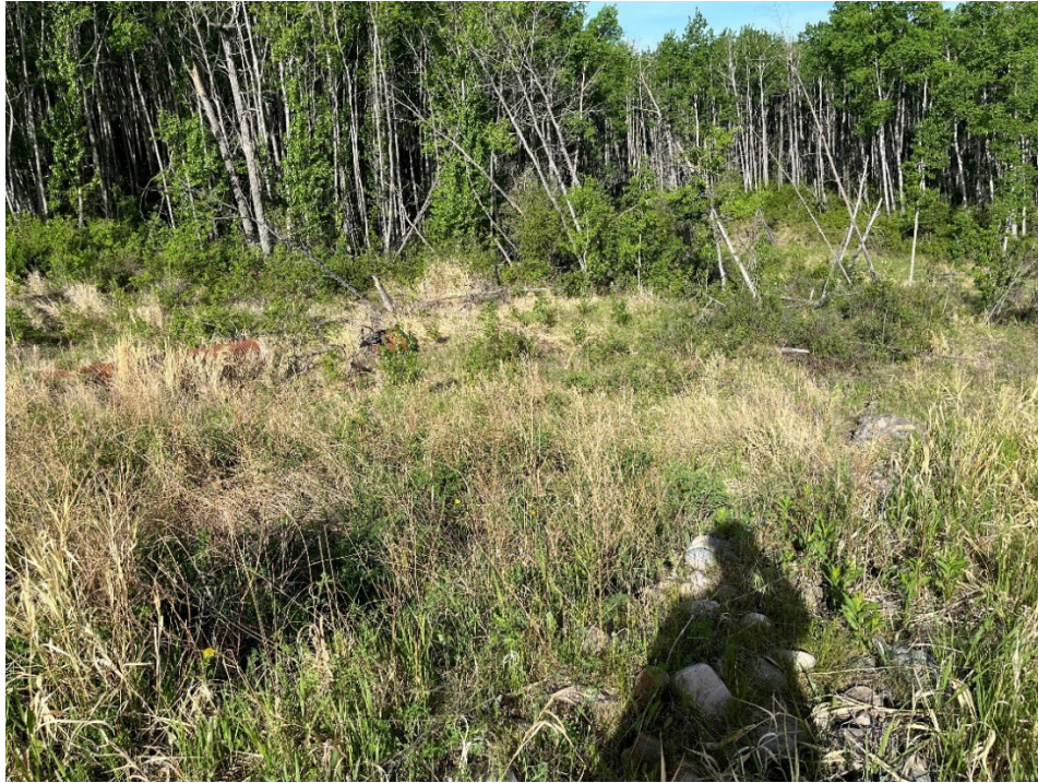
Photo 21 – Looking west where slide at km 14.45 cuts into the gabion basket swale. There has been a lot of vegetative growth in this area.
