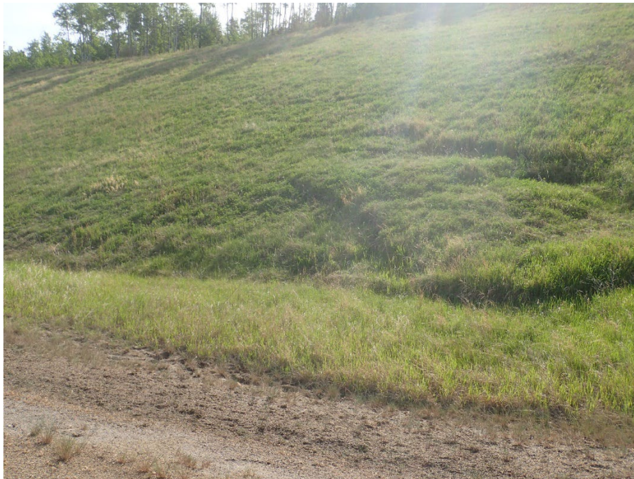
Photo 4 – Looking northeast at slump adjacent to the north gully on the lower part of the slope.
