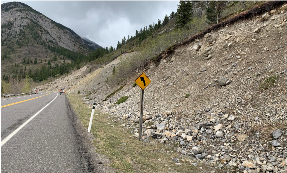
Photo 6 S070-III: Northbound ditch and bedrock fracturing. Photo taken facing east on May 9, 2023.
