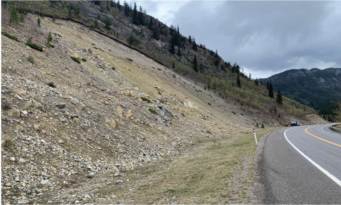
Photo 4 S070-II: Rockfall debris close to the road. Photo taken facing southeast on May 9, 2023.
